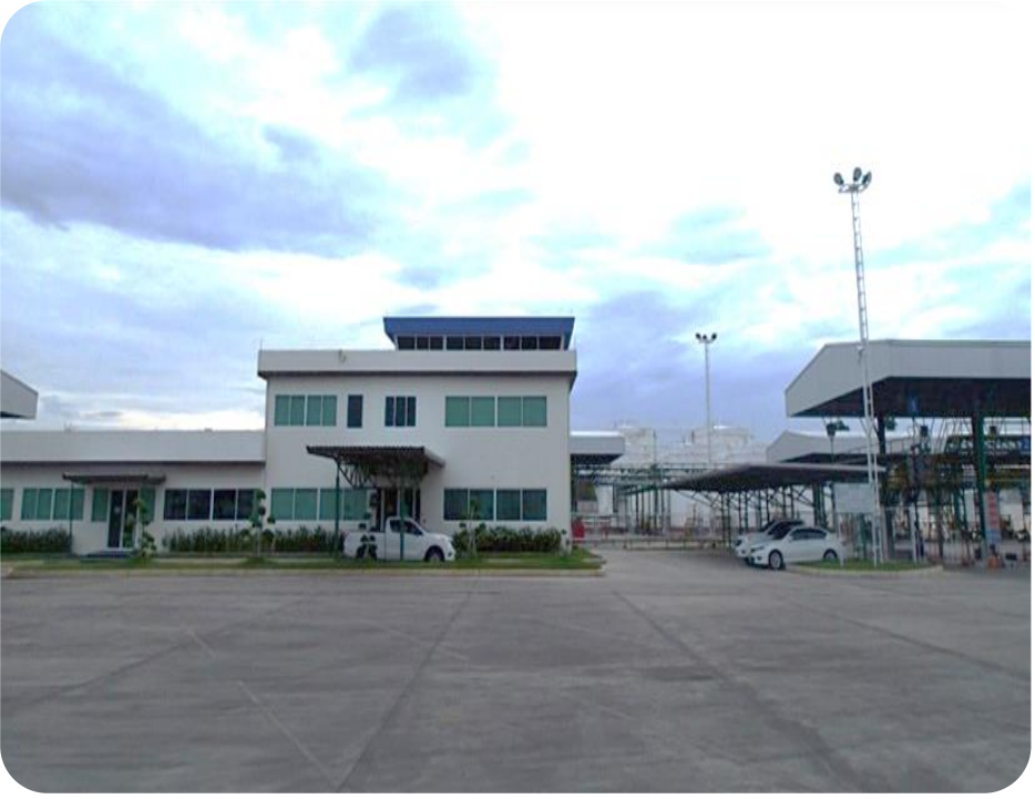
Office and Control Building
