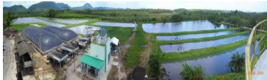
Electricity Power from Biogas
