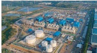
Gas-fired Power Generation
